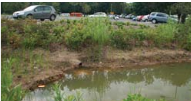
Swale to collect rainwater runoff from a new car park in Leatherhead ©Rod Shaw, Mole Valley District Council
