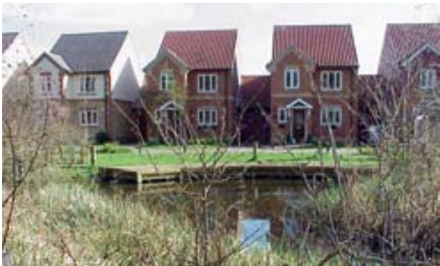
Sustainable Urban Drainage System (SUDS) – Hoebrook Close, Woking © Woking Borough Council
