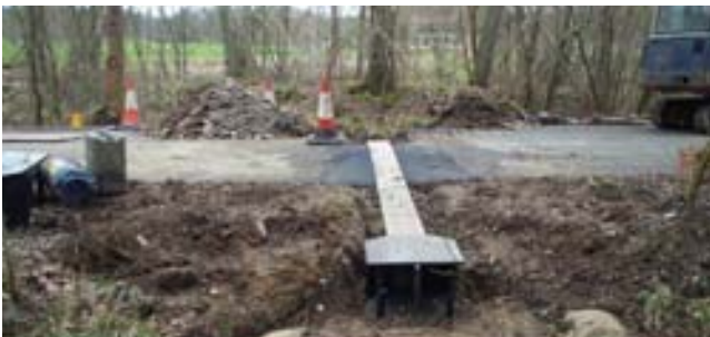
Toad Tunnel at The Drift, East Horsley. Fencing helps direct toads to the tunnel entrance © Surrey County Council
