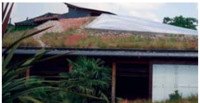
Living roof on the Komodo Dragon House, London Zoo – designed specifically for biodiversity. © livingroofs.org
