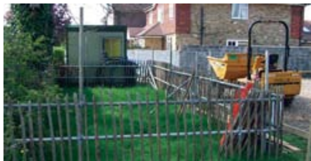
A good example of good protective fencing around a tree. The fence needs to be maintained during the life of the development to prevent damage. © Jason Hasaka / Guildford Borough Council
