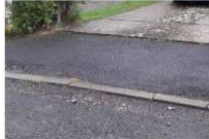
Damaged, missing or loose kerb causing a trip hazard under 2cm high
