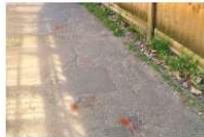
Pothole in pavement shallower than 2cm
