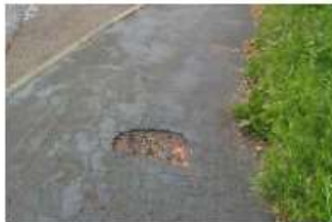
Pothole in the pavement deeper than 2cm and wider than 10cm
