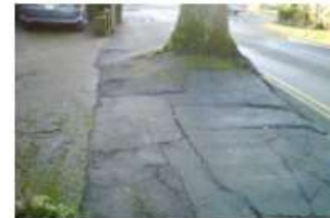
Roots causing hazard on pavement
