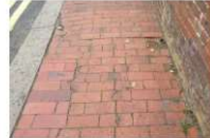
Broken, missing or loose paving or cobbles causing a trip hazard under 2cm high
