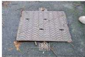
Loose or damaged manhole cover or drain causing a trip hazard on the pavement
