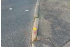
Damaged, missing or loose kerb causing a trip hazard higher than 2cm
