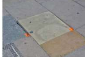
Broken, missing or loose paving or cobbles causing a trip hazard higher than 2cm
