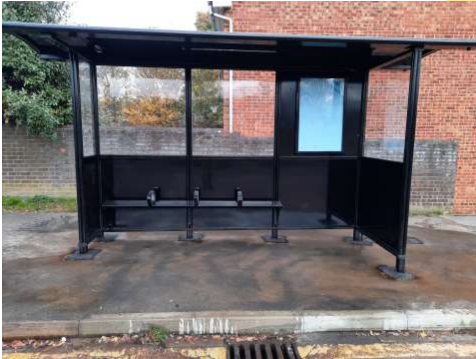
A new bus shelter installed at the Roffords stops on Marston Road, Goldsworth Park.
