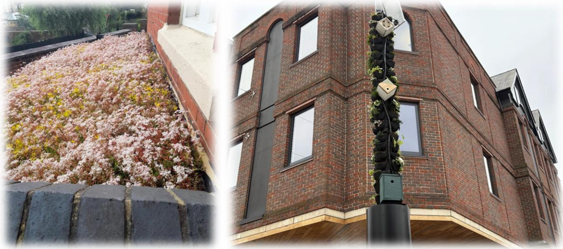
Green roof at Guildford Nursery School (left) and Living Pillar on Guildford High Street (right).
