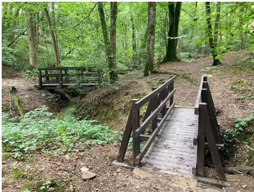
Sleeper bridges replaced by new bridges
