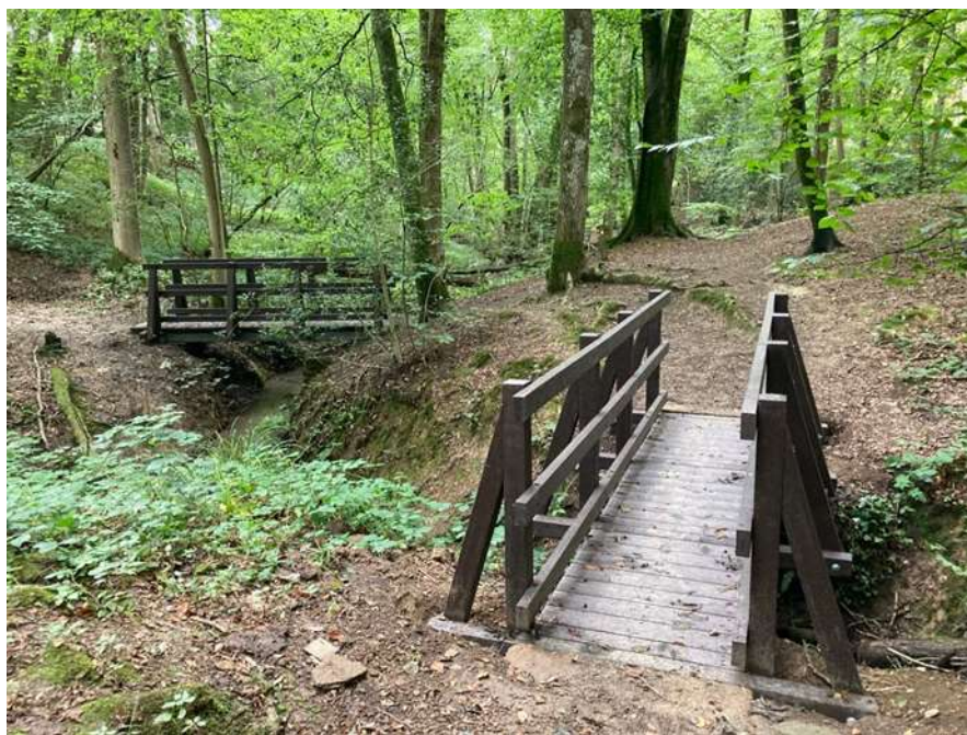
Sleeper bridges replaced by new bridges
